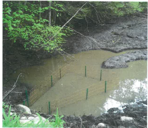
Figure 3. An exclusion fence applied to the inlet of a road culvert.
